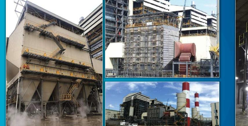
**Cenapro Incorporated** 6,600 CMH Pulse Jet Bag Filter Dust Collector
