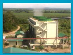
COOLING TOWERS 3 Cells x 10,000 GPM (Biscom)
