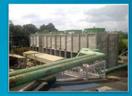
COOLING TOWERS 4 Cells X 10,000 GPM (Lopez Sugar)
