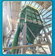
Masinloc Power Partners Co. Ltd.Republic Cement (RCBMI) - Batangas5,000 CMH Dust Collector for Roller Press Project5,000 CMH Dust Collector for Roller Press Project
