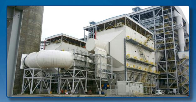
With an Electrostatic Precipitator (ESP), direct high voltage is applied to create a corona discharge to charge particles suspended in the gas and collect them through electrostatic attraction. An ESP is useful in removing particles in the sub-micron range which are difficult to capture with gravitational or centrifugal force.
